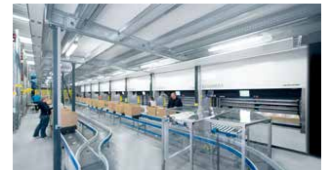
8 LogiMats are used for the picking and storage of the articles. The SSI Auto-cruiser handles the integration with the other storage areas.
