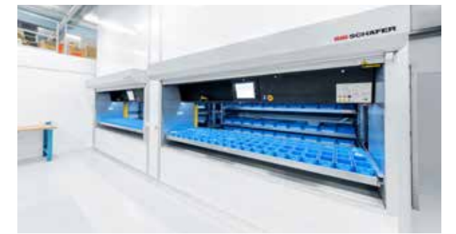
The operating opening of the vertical lift modules is located on the "main level" of the warehouse, while the vertical lift modules themselves were installed extending from the basement floor to just below the hall ceiling.
