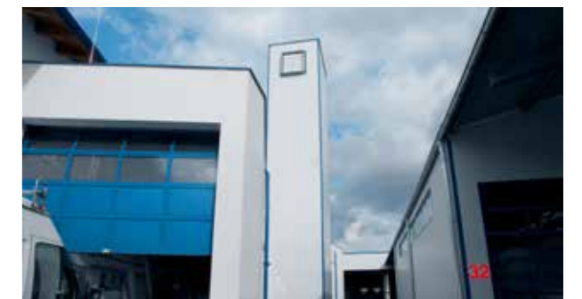
Because of the surrounding vehicle infrastructure, the LogiMat was constructed against the outer facade of the warehouse and outfitted with paneling.
